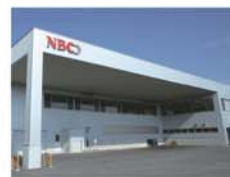
Shizuoka Kikugawa Factory
